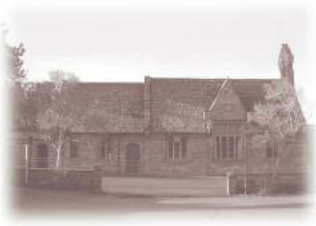
Mudford Village Hall is a Grade 2 listed building, registered charity no.292596.
